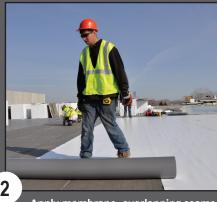
Apply membrane, overlapping seams in the direction of water run-off.
