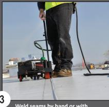
Weld seams by hand or with robotic welder.
