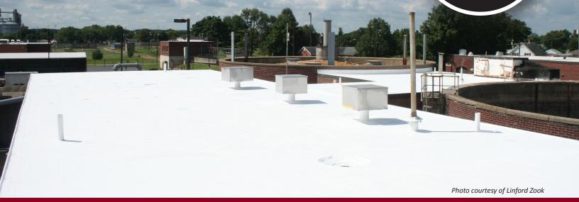
Highly reflective "cool" roofs are having their day in the sun. During the warmest weather, studies have indicated that they lower roof temperatures by up to 40% and decrease the amount of heat transferred into a building's interior. That helps reduce energy needs for cooling, and using less energy not only saves money, it also reduces the amount of pollutants released into the atmosphere. Conklin Roofing Systems meet the very highest standards for energy efficiency.
